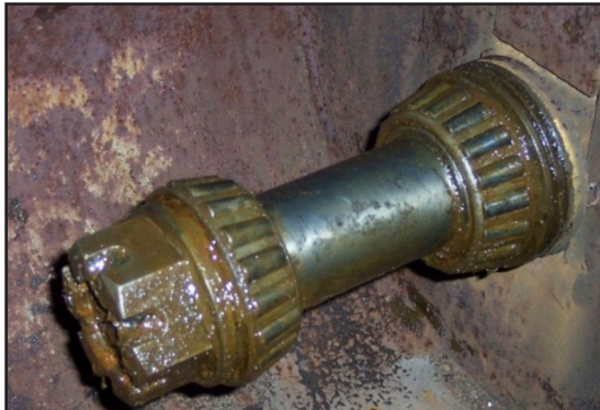
Bearing inspection revealed poor condition.
